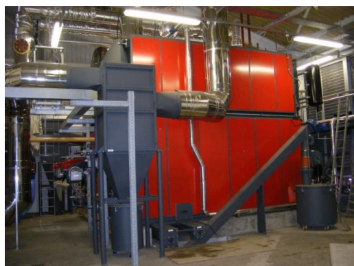
Wood boiler at the University Hospital of South ManchesterSource:AcronAPS)
